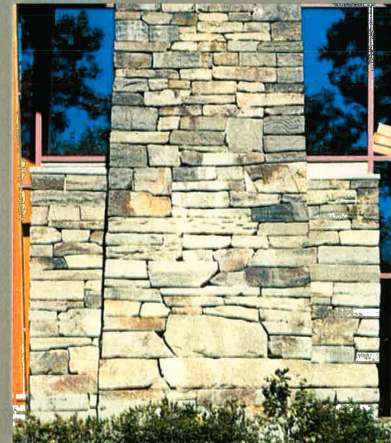
Fig. 7 A wall using a hierarchy of stone sizes.
