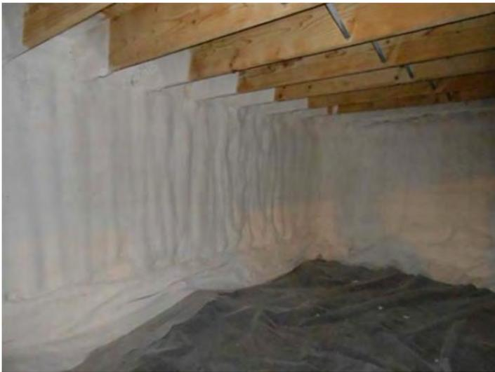
**Outstanding Insulation/Air sealing in Crawl Space**
