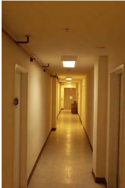
Same Hallway with Fixtures Delamped (18 FC)
