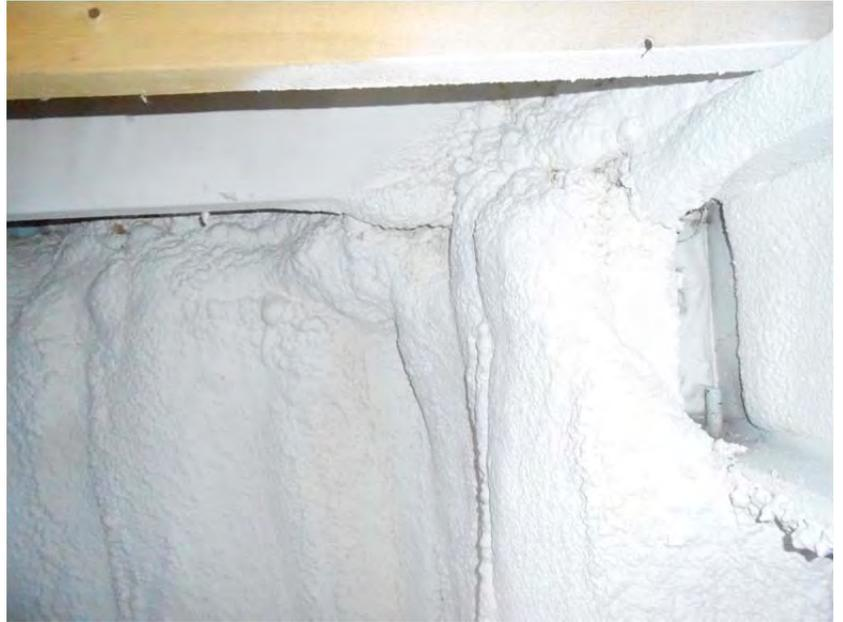
Typical Spray Foam Insulation in Crawlspace
