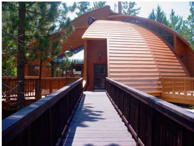
Figure 13—Copper roof on Chilao Visitor Center, Angeles National Forest.
