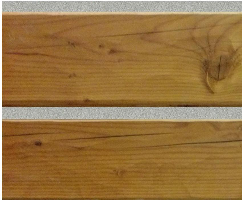
Main Siding Material – 2x12 Doug Fir Horizontal Plank Siding with Chink Line
