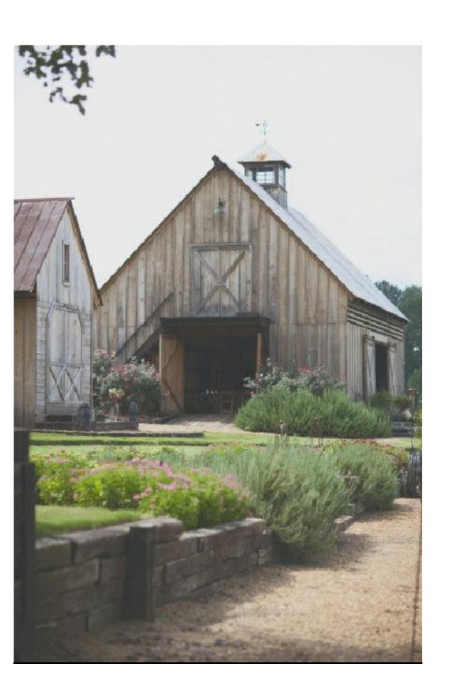
Board and batton w/ metal roof
