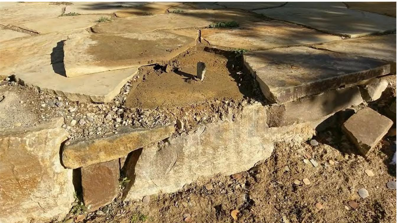
No concrete structure beneath the sand-set flagstone patio in the GE
