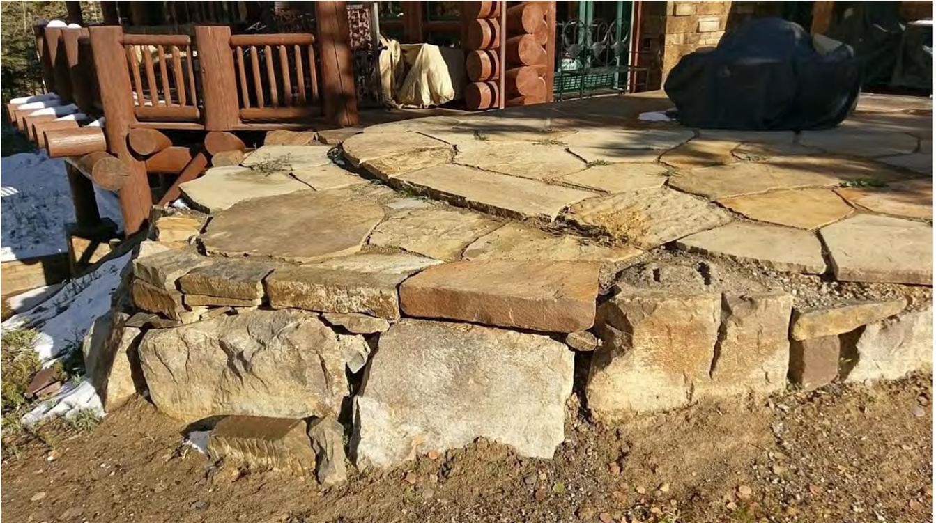
Boulder retaining at the north end of patio was added to mitigate steep slope
