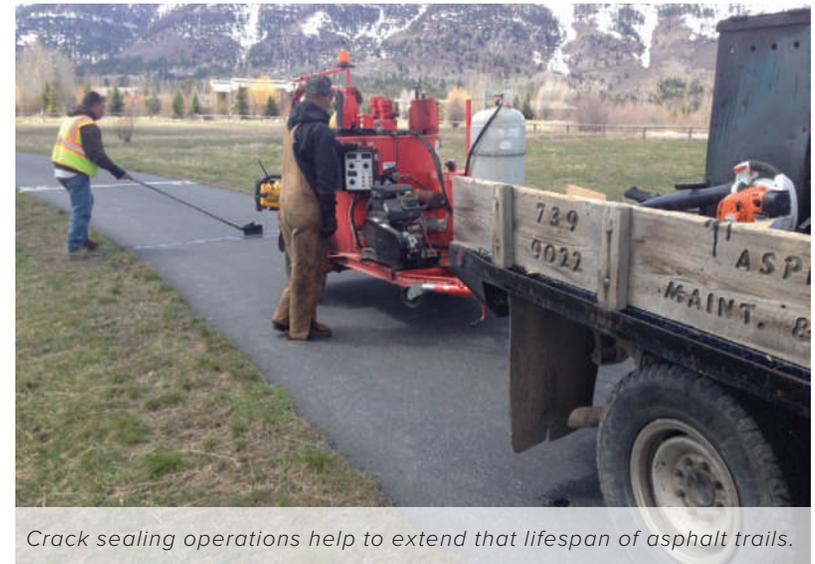
*Crack sealing operations help to extend that lifespan of asphalt trails.*
