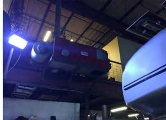
Photo #2: Waste oil heater located in Repair Garage that serves the Upper Level
