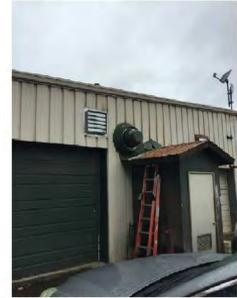
Photo #4: Repair Garage vehicle capture exhaust fan and general exhaust discharge
