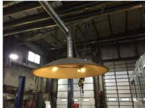
Photo #7: Repair Garage welding hood
