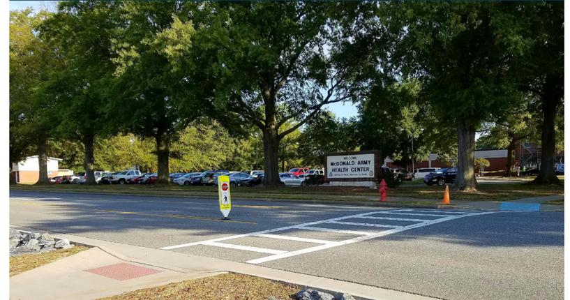
*Crosswalk improvements can include pavement striping, curb ramps, striping, signage, and flashing beacons, among others.*
