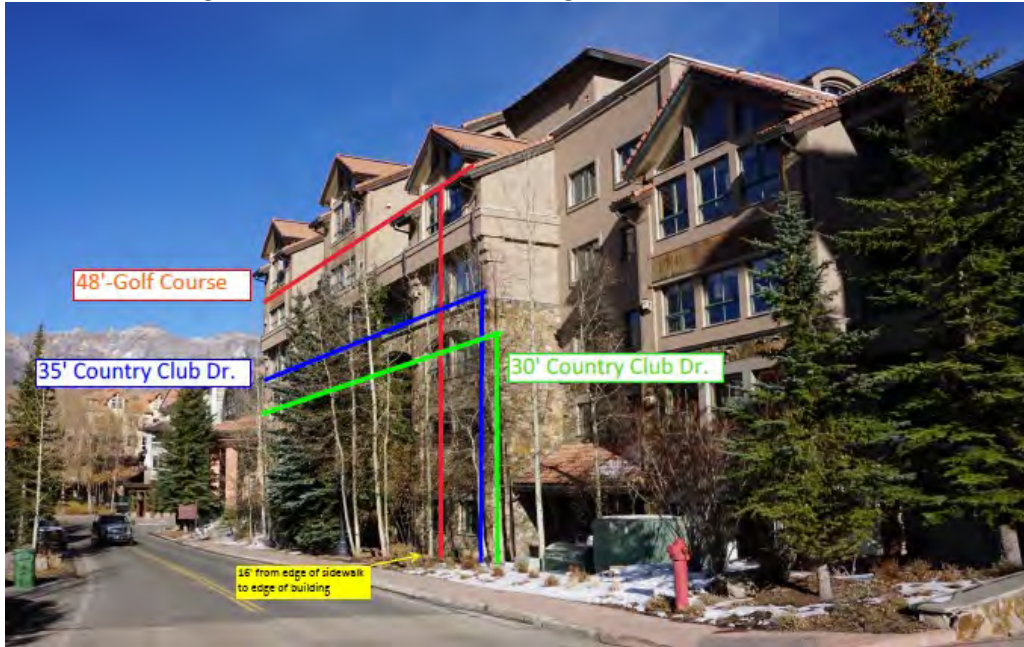
Klammer Building Viewed From Mountain Village Blvd.
