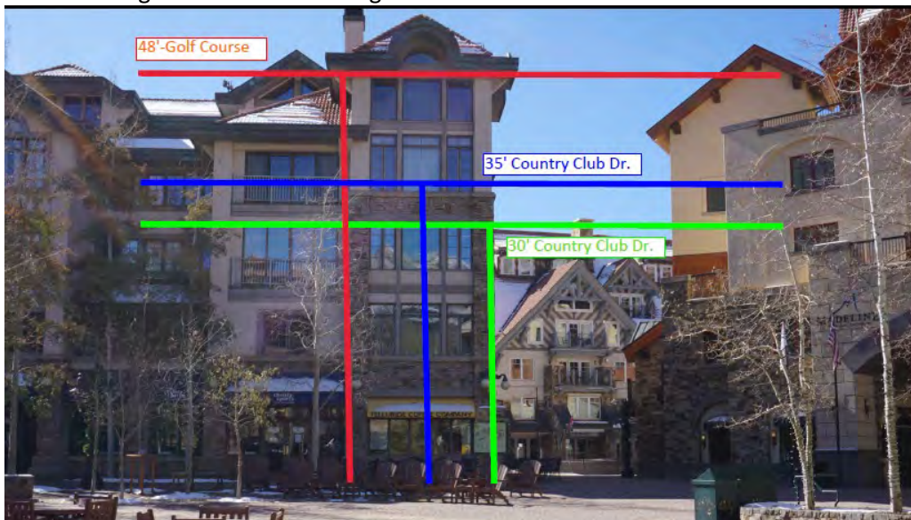
Plaza Building Viewed From Heritage Plaza
