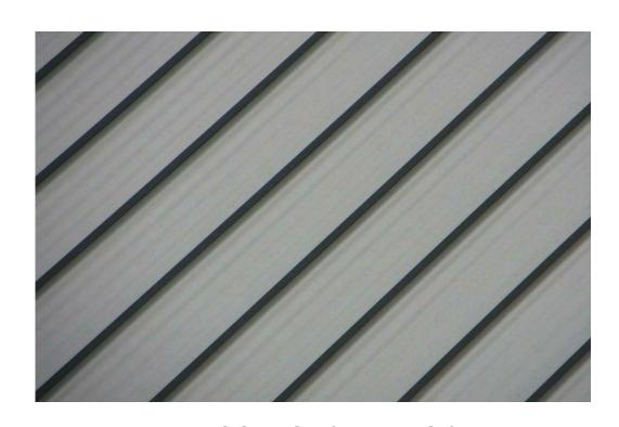
NEW METAL ROOFING - STANDING SEAM
