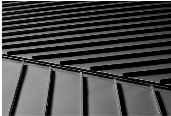
M1 - ROOFING / SIDING - STNDING SEAM 16" O.C.
