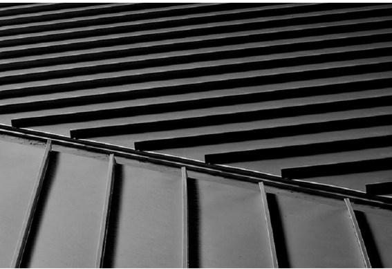
M1 - ROOFING / SIDING - STNDING SEAM 16" O.C.
