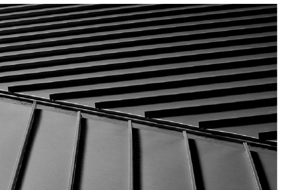
M1 - ROOFING / SIDING - STNDING SEAM 16" O.C.
