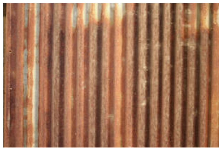
RUSTED STEEL CORRUGATED ROOFING
