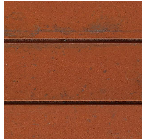
RUSTED HORIZONTAL STEEL SIDING
