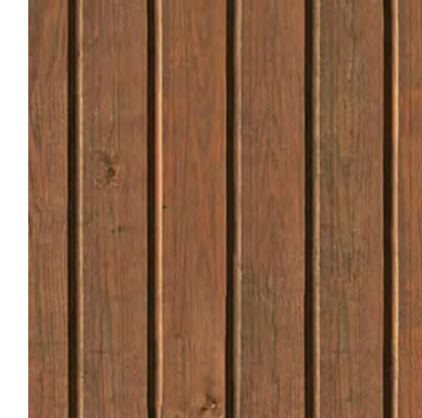
VERTICAL WOOD SIDING: 6" DOUG FIR VERT SIDING W/ MITERED CORNERS
