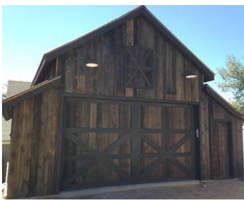
VERTICAL WOOD SIDING: 8" MILLCREEK TELLURIDE STONE GREY BARNWOOD SIDING W/ MITERED CORNERS FINISH: TYPICAL STAIN
