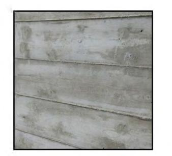
**EXPOSED CONCRETE: BOARD-FORMED**
