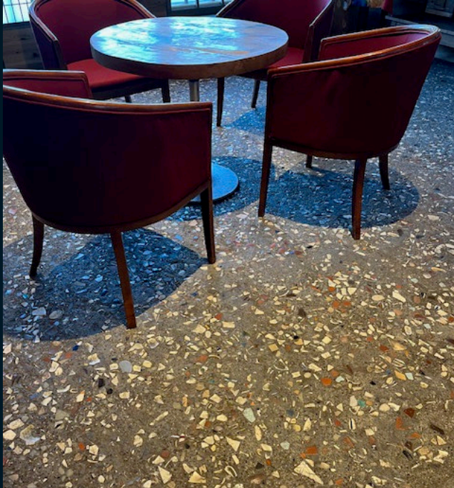
Concrete floor made from crushed ceramics
