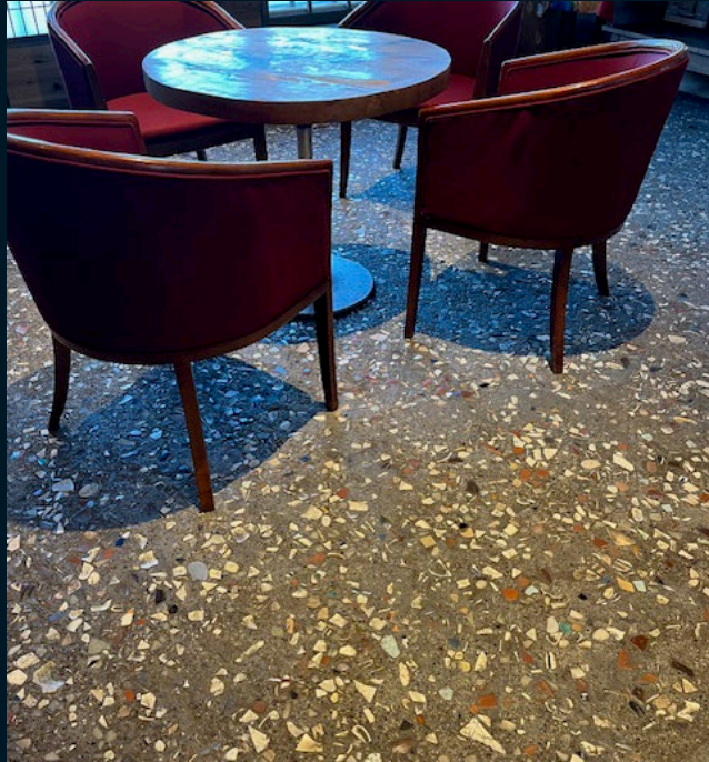
Concrete floor made from crushed ceramics
