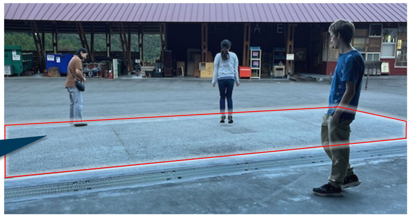
A built-in scale weighs trucks before and after being filled. The community tracks on the collection data.
