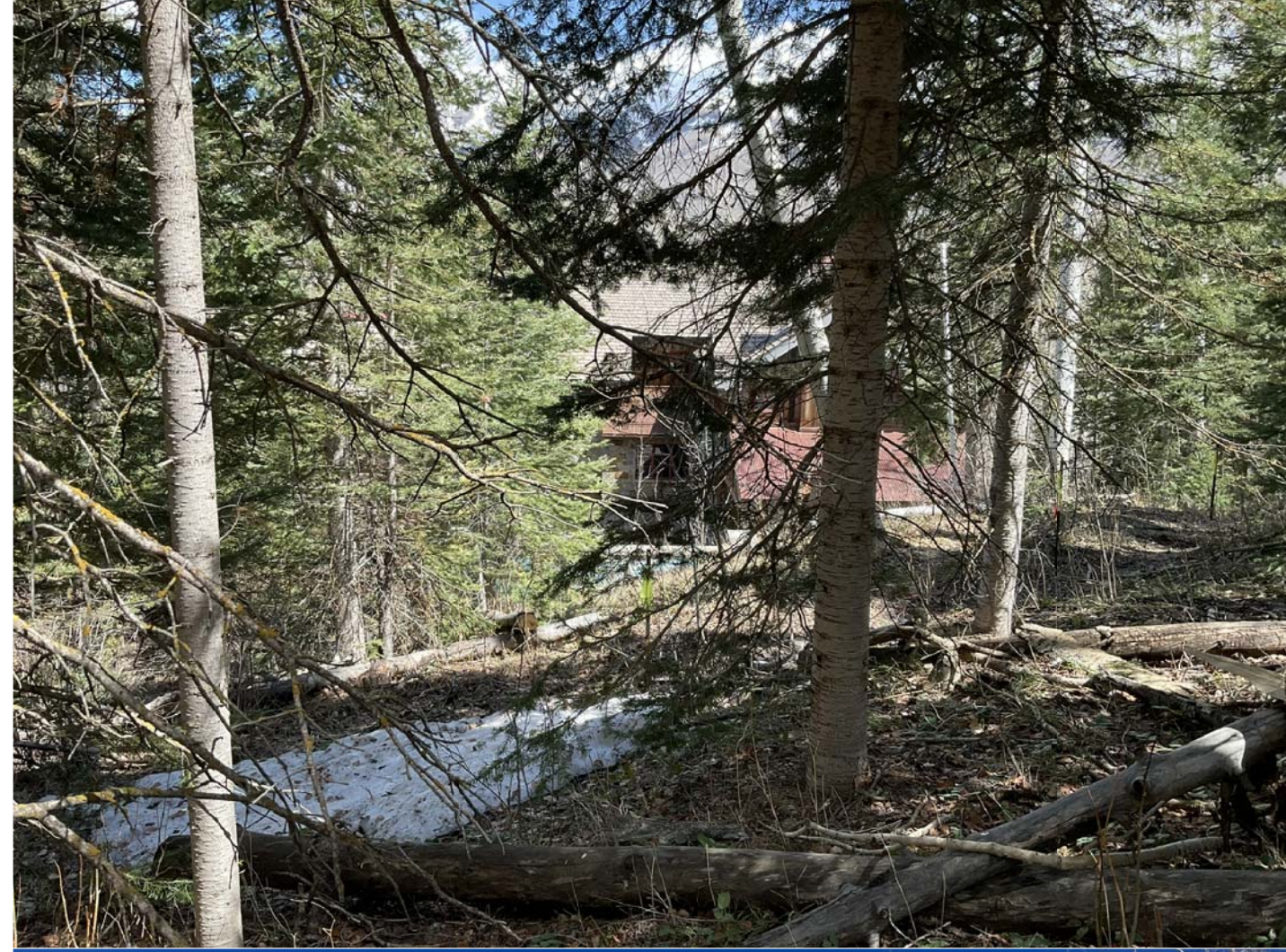
ENTRY STAIR LOOKING NORTH
