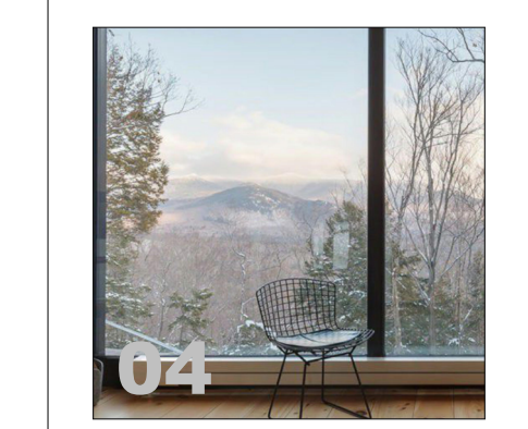
04 GLAZING: High energy double-pane low-e glazing
