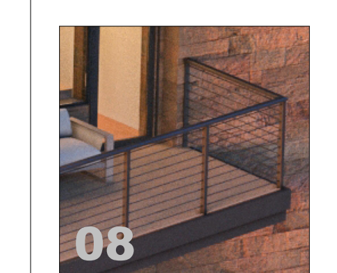
08 RAILINGS: Cable railing with 2x2 metal balusters
