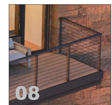
08 RAILINGS: Cable railing with 2x2 metal balusters
