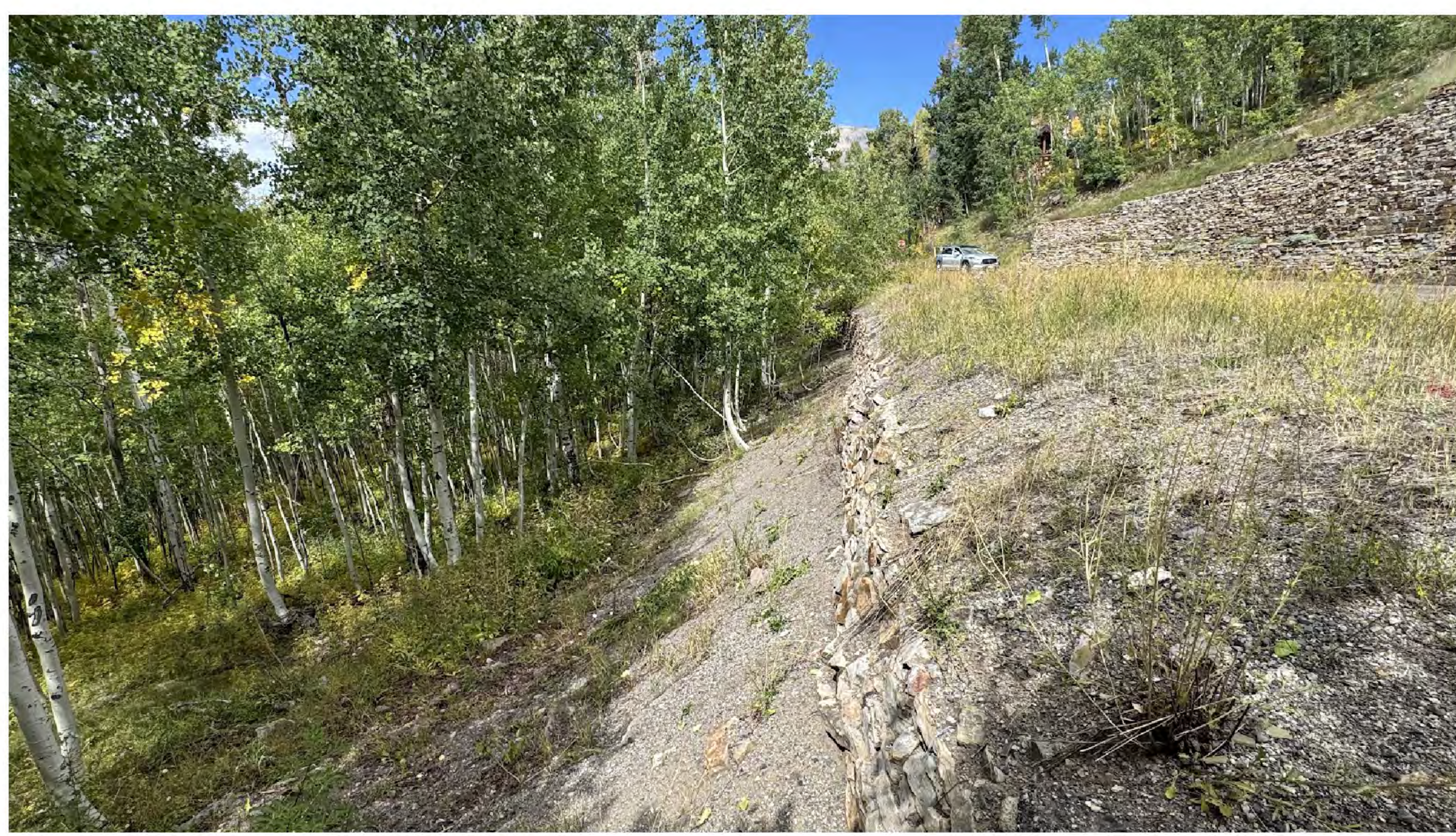
VIEW OF LOT SHOWING RETAINING WALL
