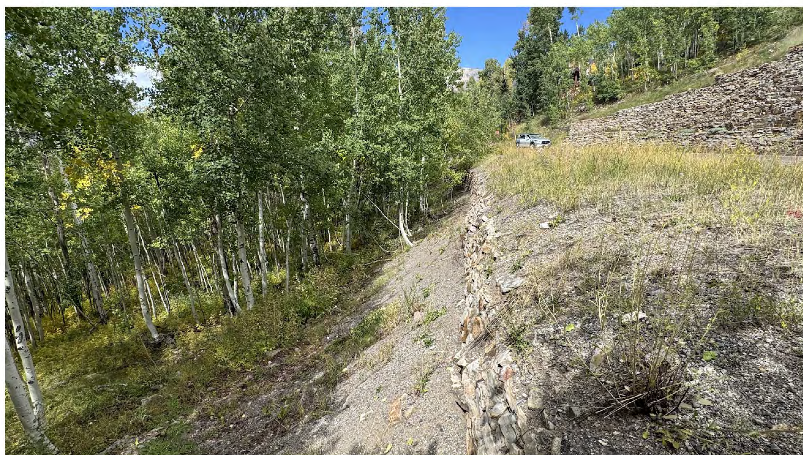
VIEW OF LOT SHOWING RETAINING WALL
