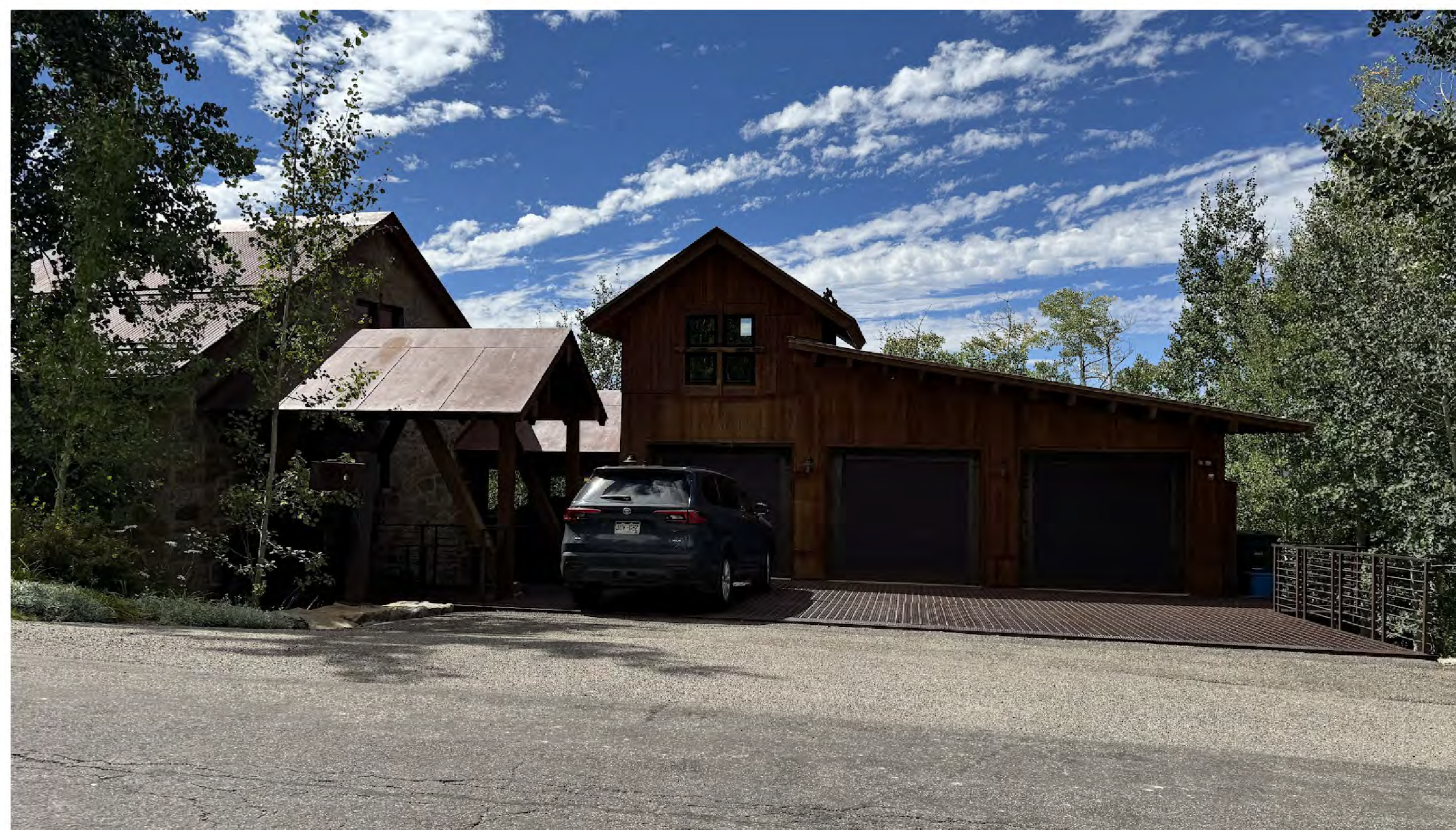
VIEW OF HOUSE TO THE NORTH
